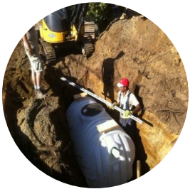
1. Rainwater Tank (Timing TBD)
