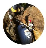
A storm water tank will be required for all multiplexes. It should generally be located underground in the front yard.
