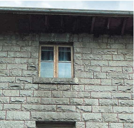
18. Soffit condition
