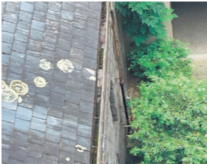
10. Roof lichen and moss in gutters
