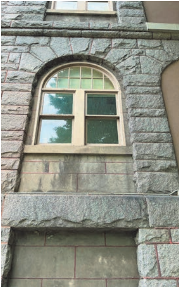
26. Concrete infill sill and new window
