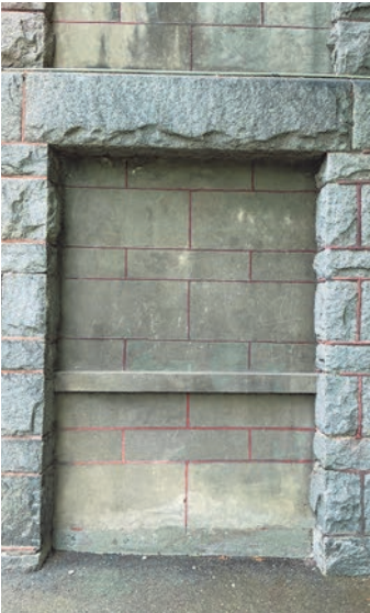
25. Tooled concrete infill
