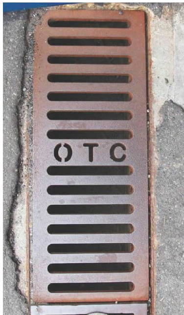
Replicated OTC Drains
