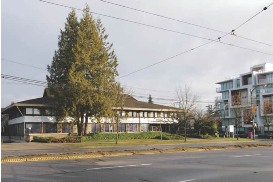
Oakmount Medical Centre on W 41 st Ave.
