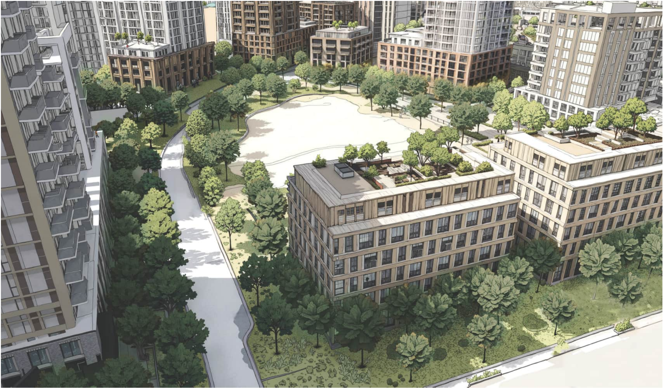
Aerial view looking South from W 38 th Ave
