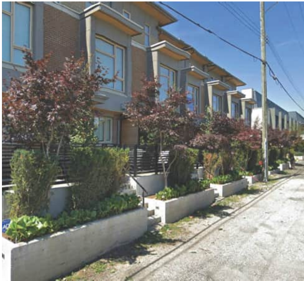
Site Photo - Existing West Lane
