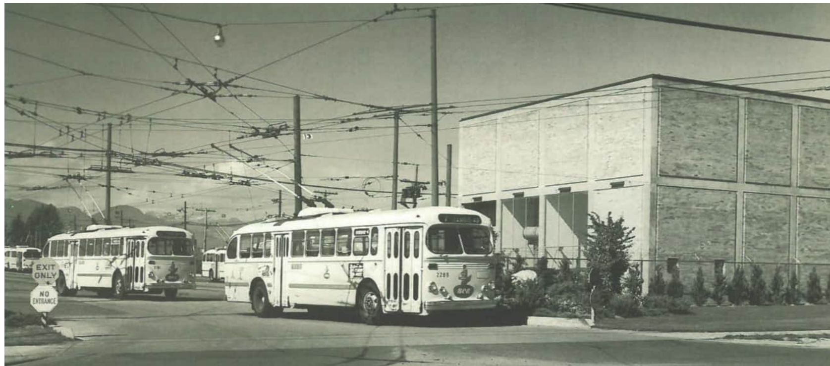
The Substation and Trolley Buses in 1955
