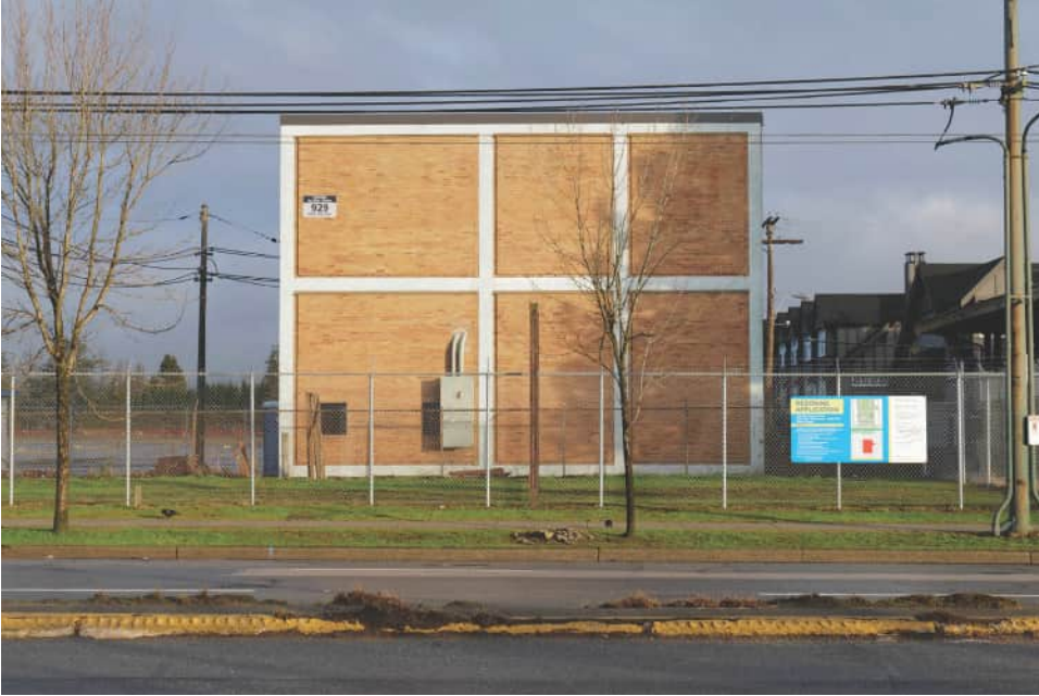
Rectifier Station on W 41 st Ave.
