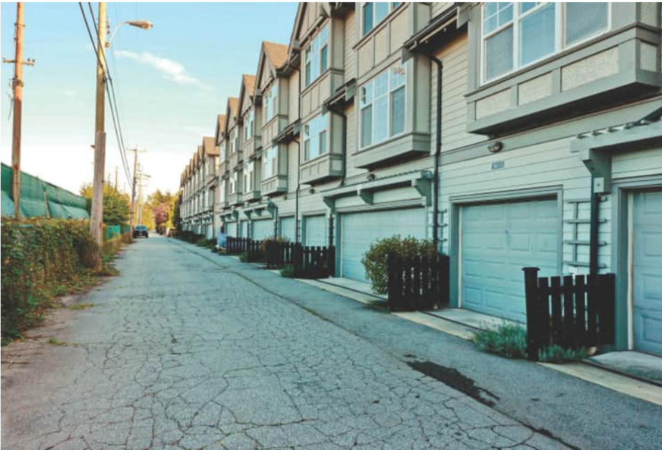
East Lane, Looking North
