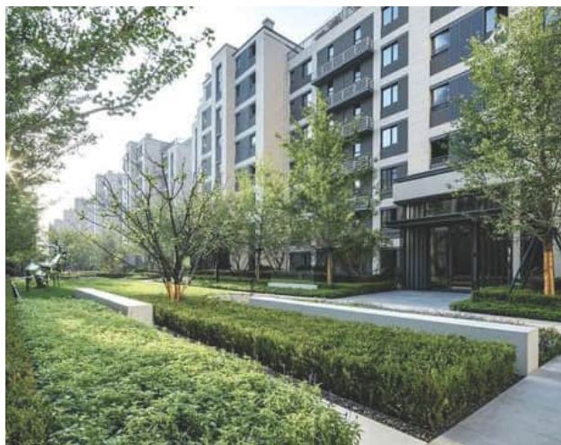
Precedent Image - Lobby Entrance
