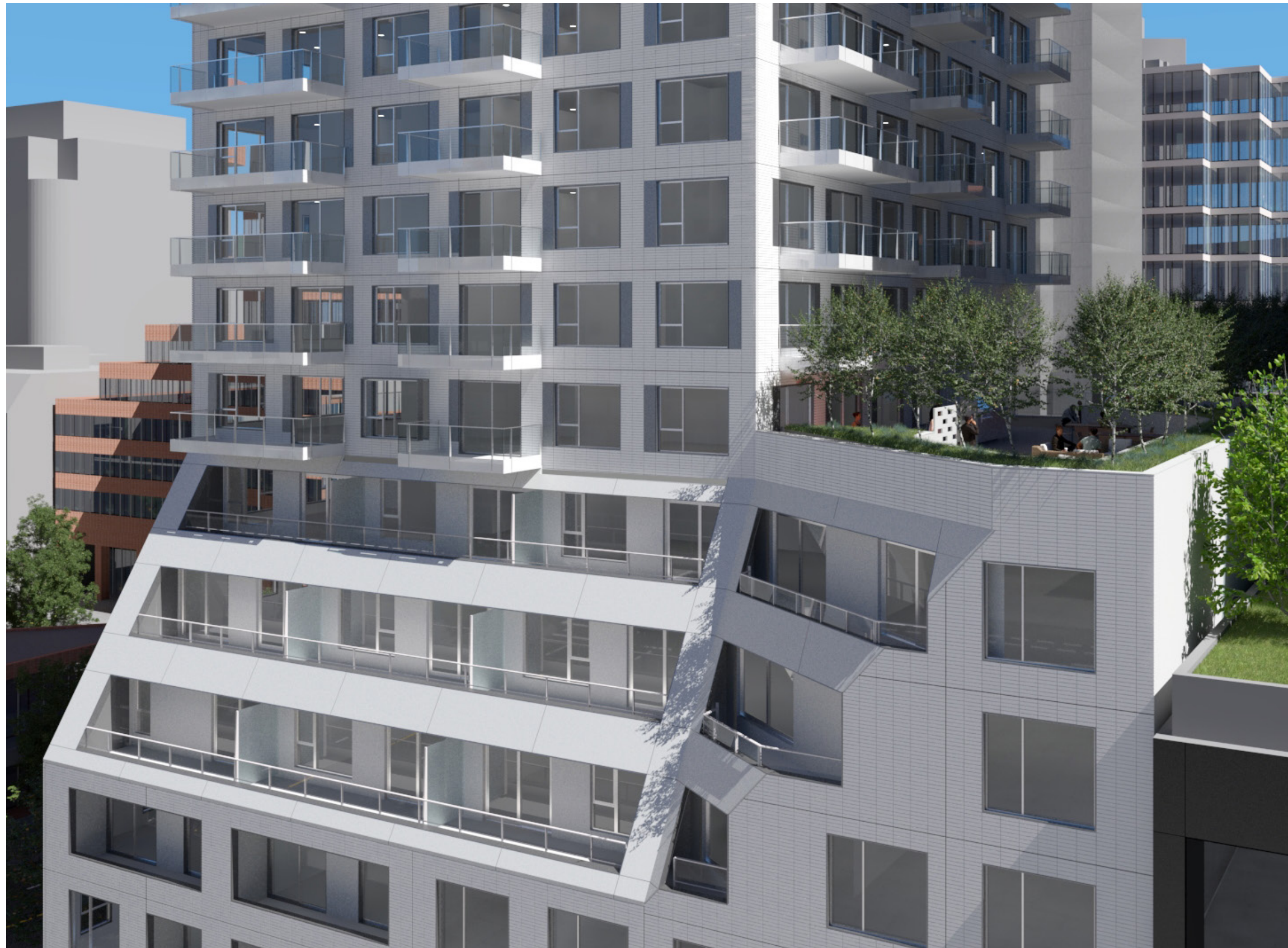
SLOPED FACADE AND TERRACES ALONG LANE EDGE
