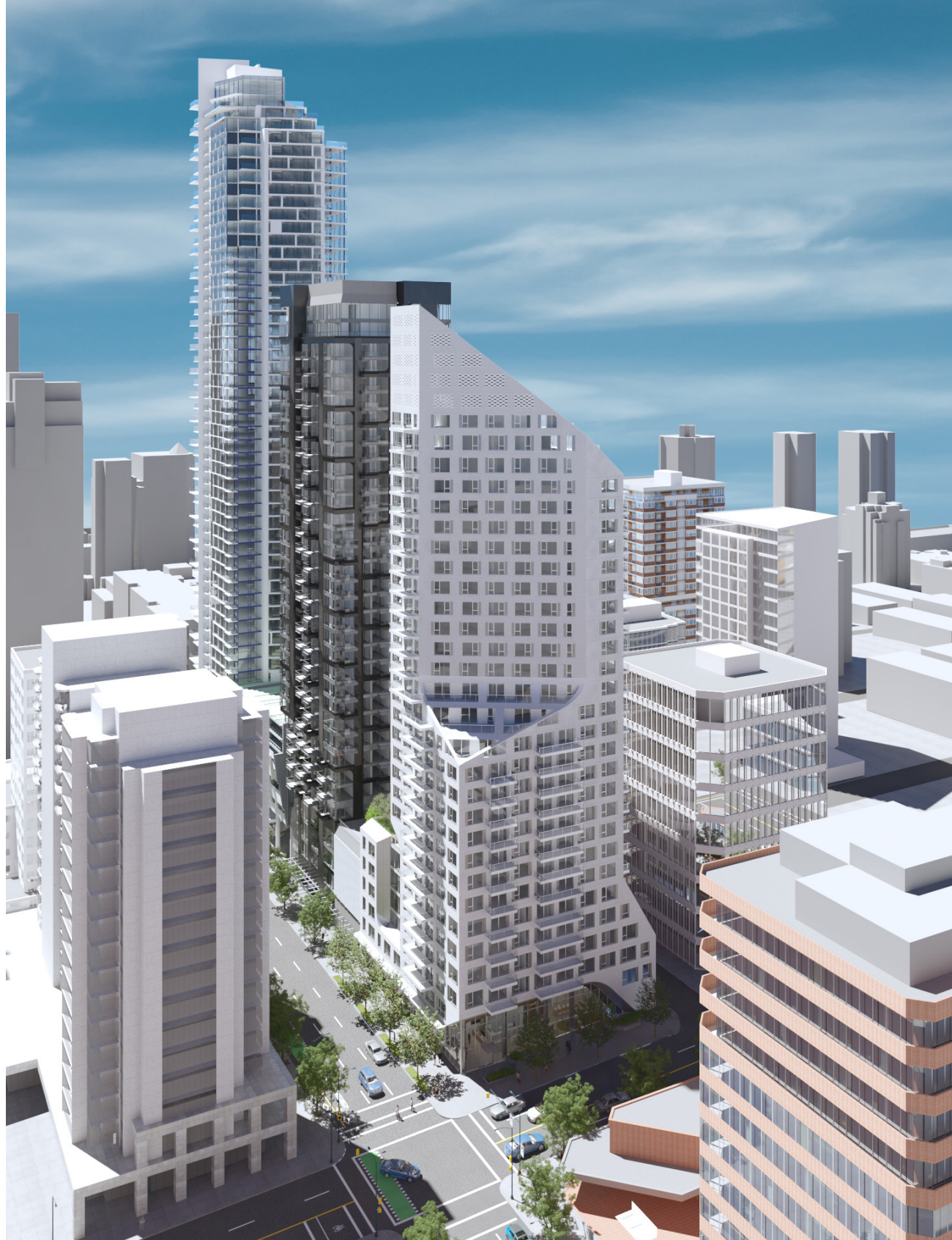
AERIAL VIEW AT THE CORNER OF HORNBY STREET AND DAVIE STREET
