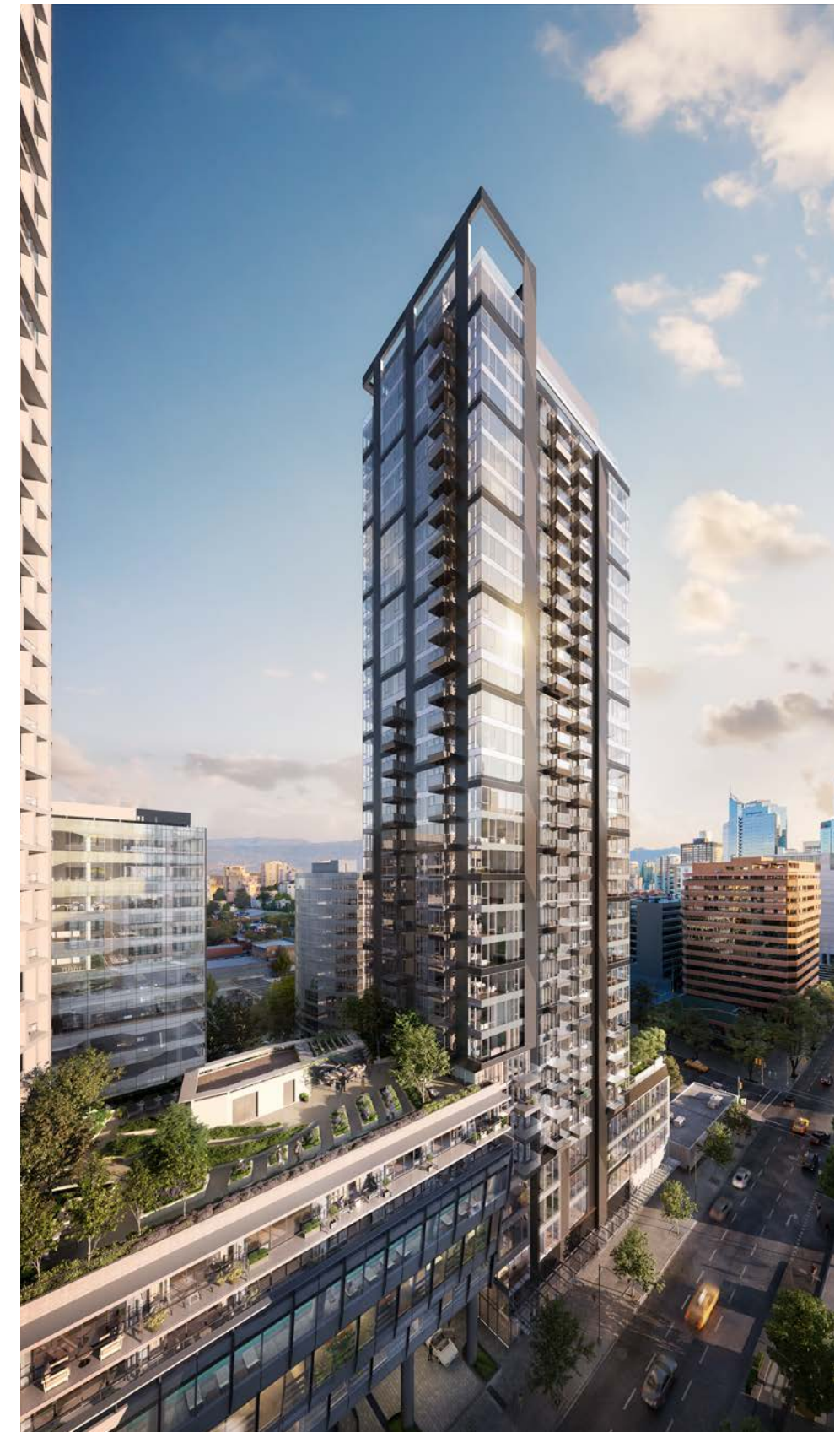
2 Burrard Place, Vancouver. Reliance Properties, NMDA + Bingham + Hill
