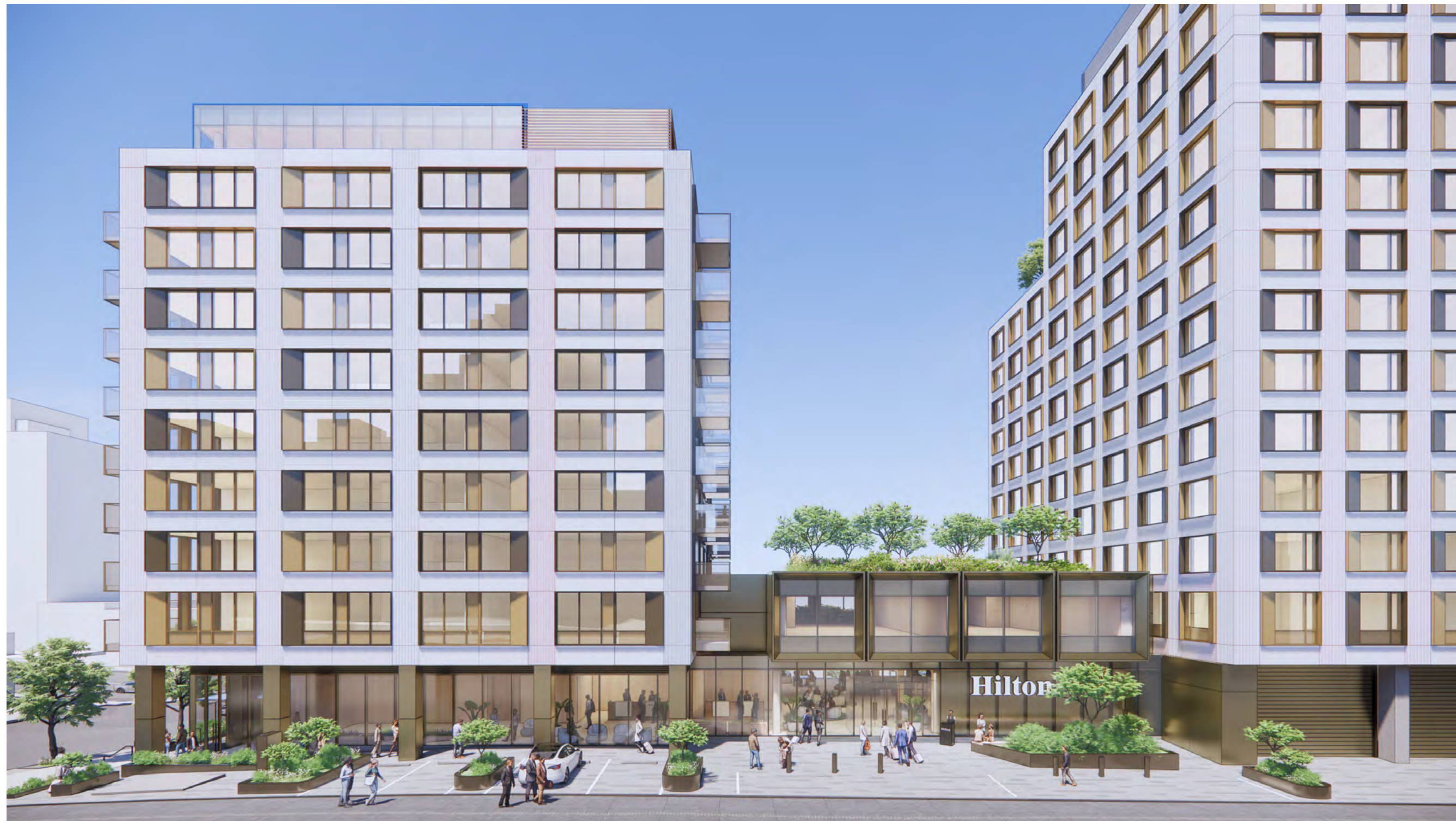
View from Lane looking North
