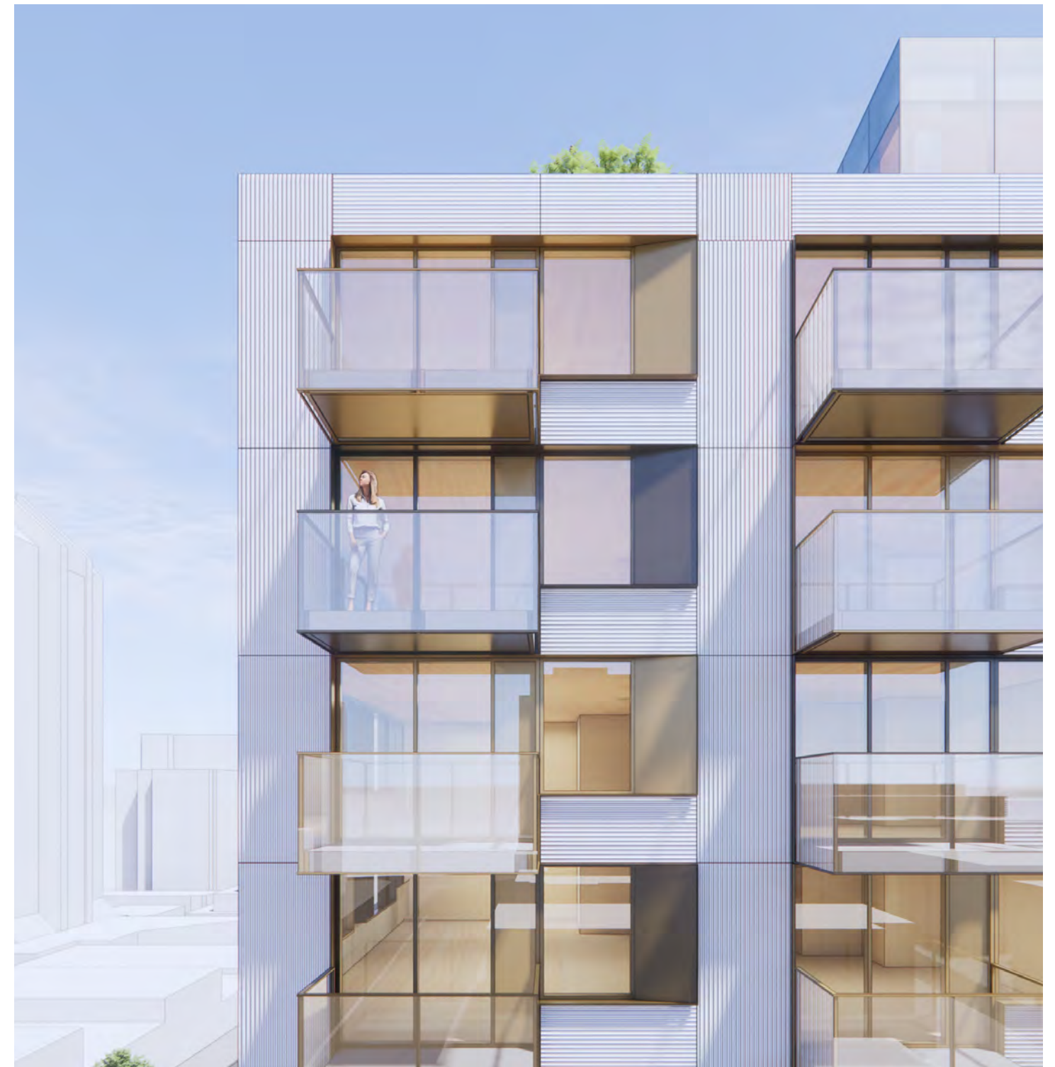
888 W Broadway – Insulated Fiber Cement Panel Design
