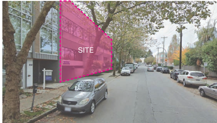
A. Looking West along W 8th Avenue
