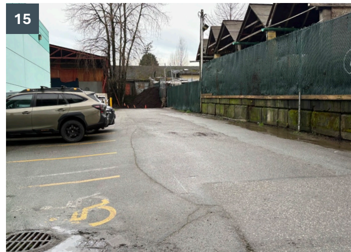
Figure 22 Southern Portion of Rear Lane Looking at Encroachment (S of the Site)
