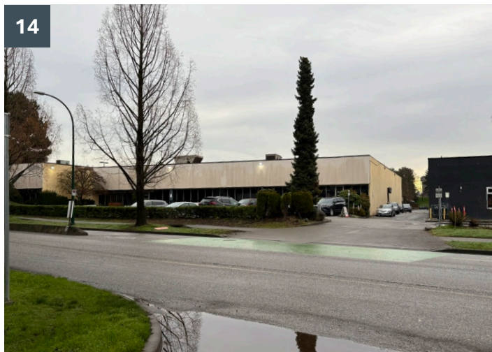
Figure 21 Manufacturing Buildings (SE of the Site)
