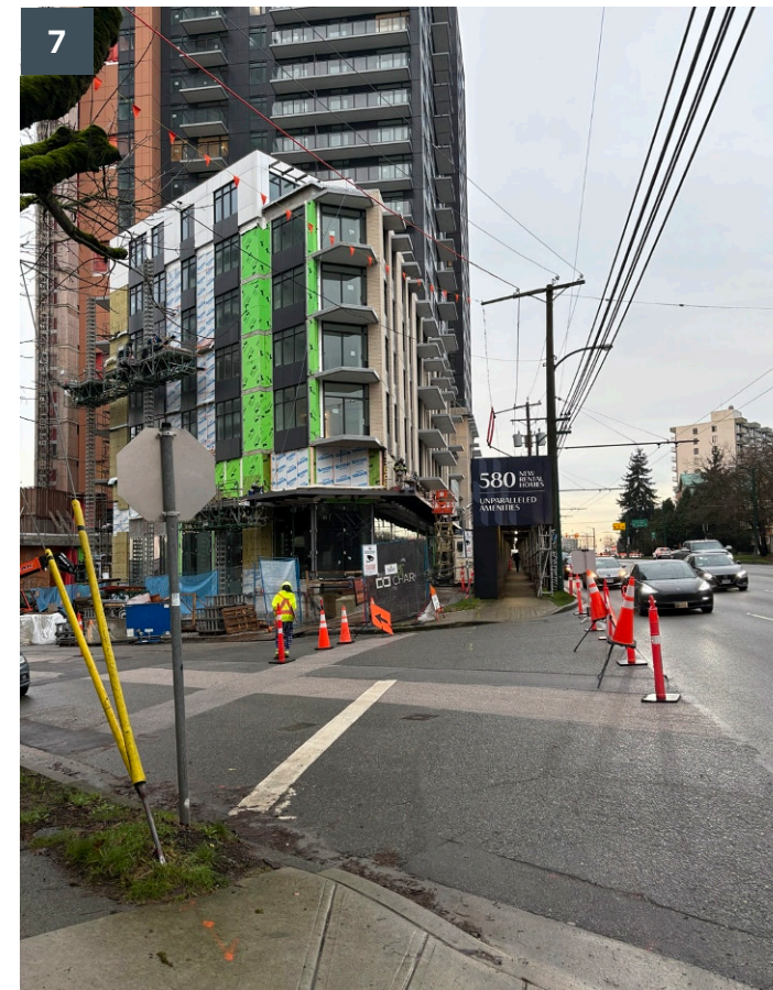
Figure 14 Mixed-Use Tower (NW of the Site)
