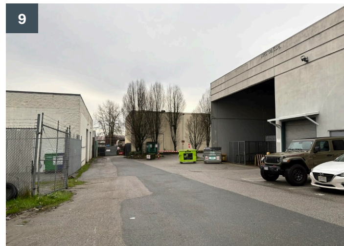
Figure 16 Rear Lane Looking at Encroachment (W of the Site)
