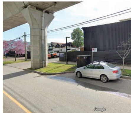
D. South West Corner: Looking west
