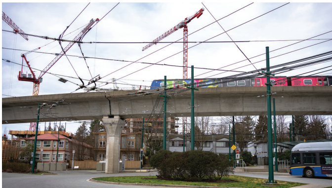
View from the Bus Loop, Facing West towards Site
