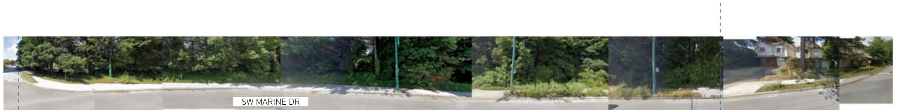
8 SW Marine Drive Elevation (Facing Site)
