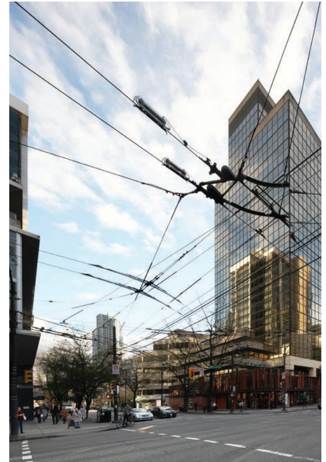
View from Robson Street at Burrard St
