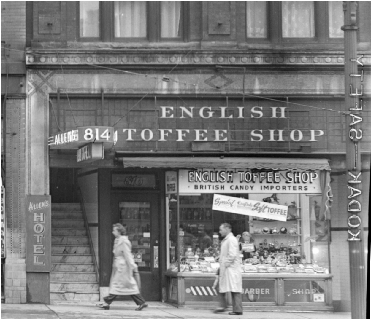
View of the Allen Rooms storefront in 1950. With the exception of the original (or very early) marquee, which was removed in the mid 1920s, the storefront remained unaltered until its renovation in circa 1951. (Artray; Vancouver Public Library 81449)
