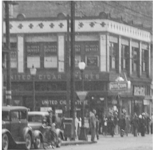
Above: View of the Service Building in 1932. Note the round, galvanized iron rounded merlons along the parapet. (City of Vancouver Archives 20-58)
