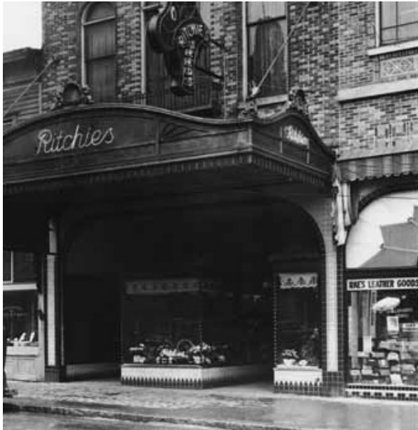
Northern most storefront with original canopy. Note adjacent storefront design and materials including original fan light transom, 1931 (1931. Thomson, S. VPL 9007)
