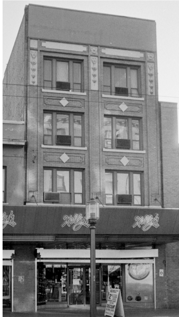
View of the front façade of the Allen Rooms in circa 1985. (City of Vancouver Archives 790-1827)
