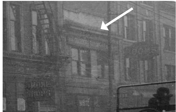
Historic view of original parapet with metal cornice as viewed from Granville Street, 1910s. [CVA Trans N87.08]
