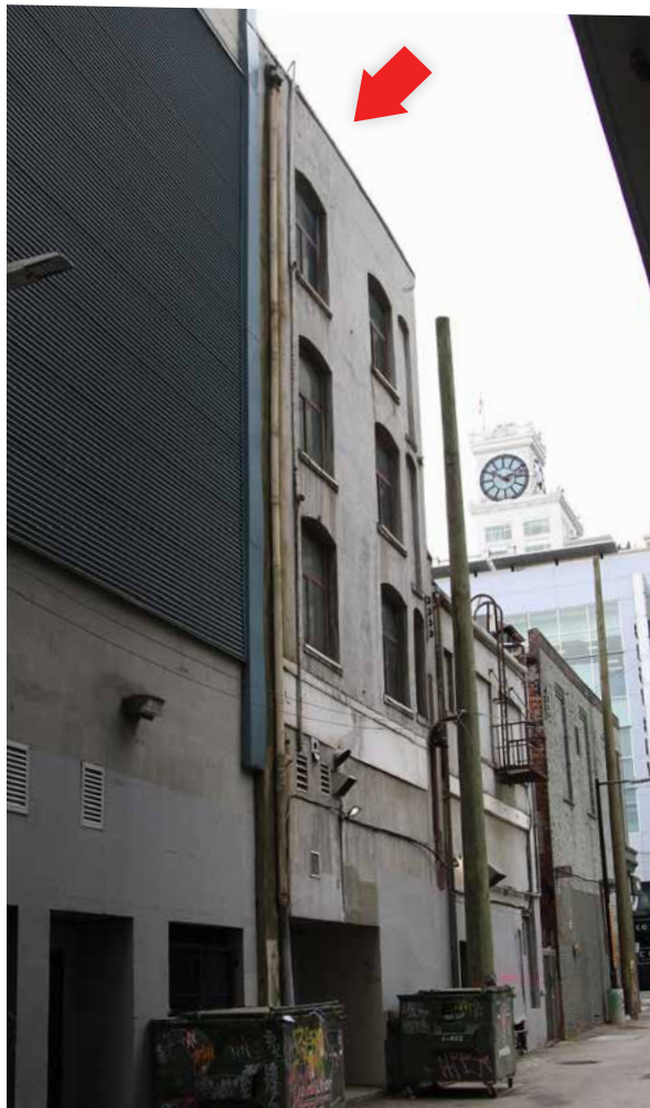
View of the rear façade of the Allen Rooms, July 2021. (Donald Luxton & Associates)
