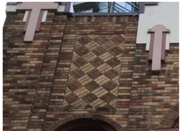
Spanish bond panels below continuous parge band and mosaic panels with header surrounds of the front façade.
