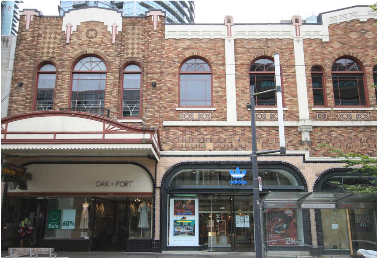
Brickwork of front elevation of the Commodore Ballroom featuring multi-coloured brick laid in running bond, triple basket weave panels (above arched windows), Spanish bond panels (above storefront), arched soldier course lintels, and header surrounds.
