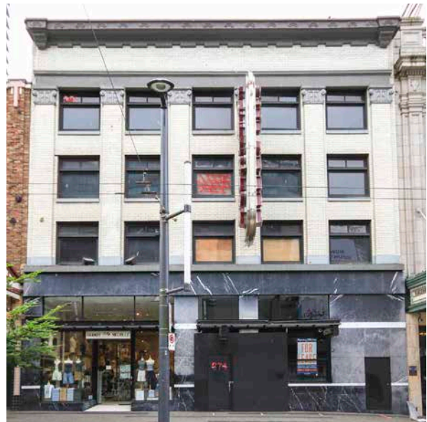
Front façade of the four-storey Norfolk Rooms, July 2021. (Donald Luxton & Associates)
