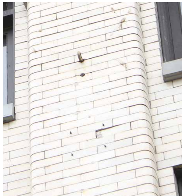
Redundant anchors still installed into brick faces and mortar joints of the front façade, July 2021. (Donald Luxton & Associates)
