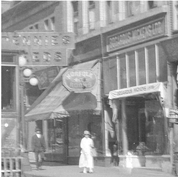
Retractable canopies, painted signs, and blade signs all affixed to the Norfolk Rooms' storefront in a circa 1920 image. (City of Vancouver Archives 1376-129)
