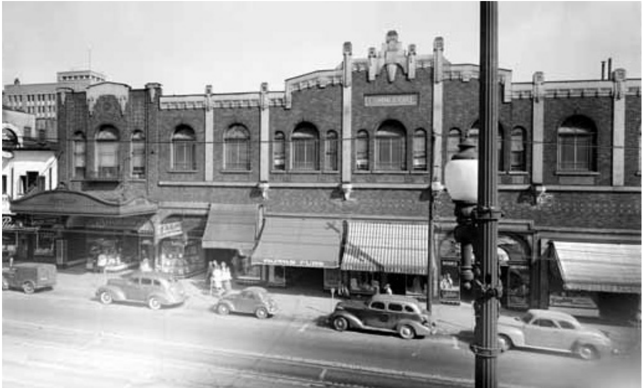
Commodore, 1950, (VPL 83192). Earliest portion built is at the far left (current entrance to Commodore Lanes), one of the early tenants in this portion of the building was a Japanese goods store - Mikado.
