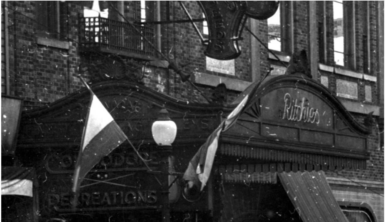
Above: Cantilevered canopy at the north end of the Commodore Ballroom with sign for basement level recreations evident (VPL 11037).
