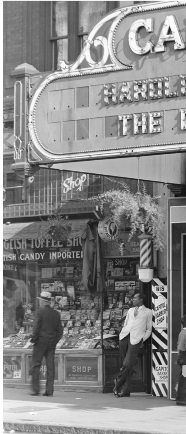
Partial view of the southern portion of the original storefront of the Allen Rooms from 1934. Note the glazing in the bulkhead to provide light into the basement, and the Luxer Prism Glass transoms above the display windows. (Dominion Photograph Co.; Vancouver Public Library 23587)
