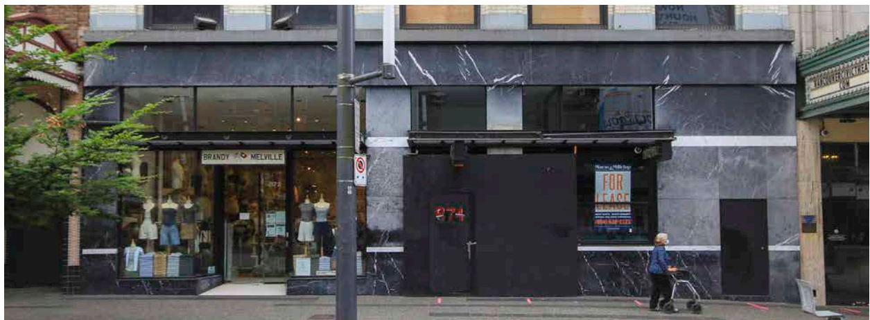
Top: Elevation drawing of the proposed new storefront in 1935 by architect Thomas L. Kerr. (City of Vancouver Archives COV-S393-1, AP-533); Middle: The storefront of the Norfolk Rooms as it appeared in 1935 following its alteration. (City of Vancouver Archives 99-4766); Bottom: The Norfolk Rooms storefront as it appeared in July 2021. (Donald Luxton & Associates)
