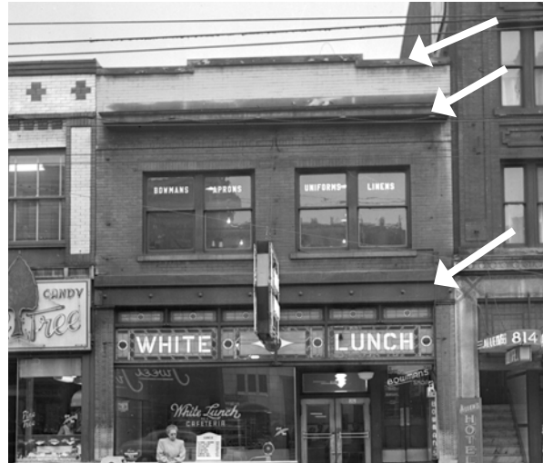
Historic view of original parapet with metal cornice and cap flashing as well as the original storefront cornice as viewed from Granville Street, 1950s. [VPL 81449]
