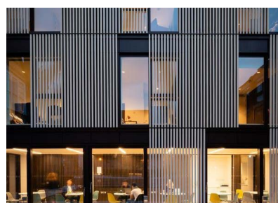
5 screens and grilles
