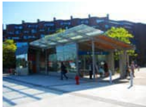
① Oakridge Transit Station
