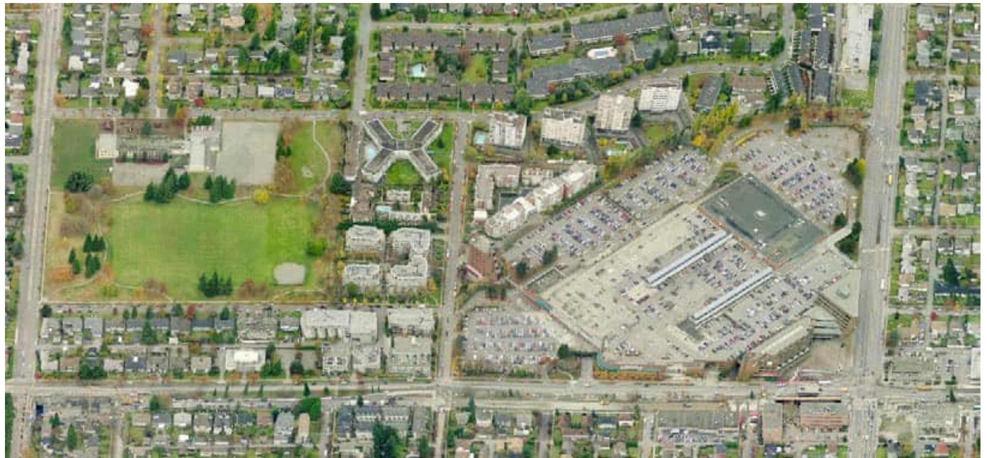
Site Aerial View (2010)
