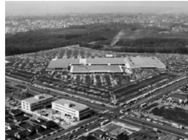
1950s construction photo
