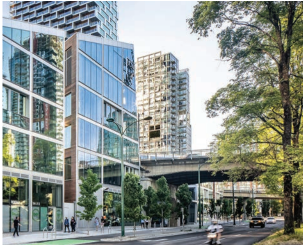
Pacific Street looking west, with the project site to the right
