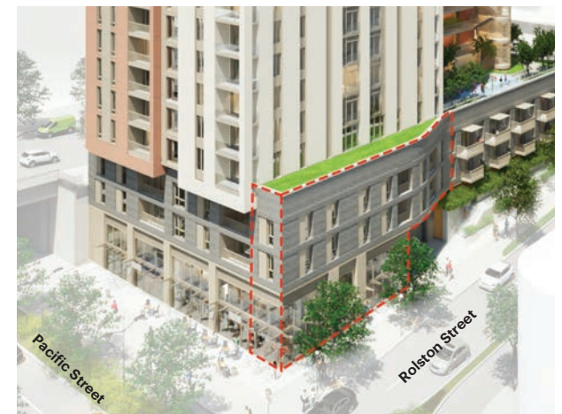
Aerial view of massing at the intersection of Rolston and Pacific Streets demonstrating how the proposed encroachment provides a setback for the tower massing along Rolston.
