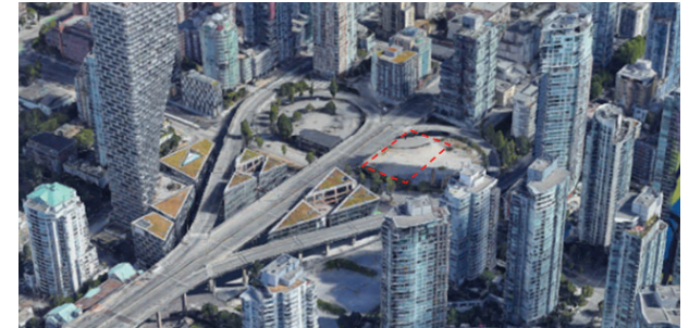
Aerial View from South (prior to demolition of the Granville Loops)
