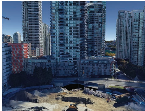
Site View Towards East (Google Earth)
