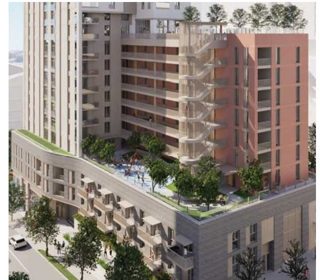
Rendered view of the proposed project, showing morning sunlight at what was proposed to be the childcare outdoor area (Level 5) in the Rezoning Form of Development, and what is now proposed to be a shared residential amenity area with a children's playground. Note that while direct sunlight access is similar to what was proposed in the rezoning Form of Development, access to view of the sky and surroundings is significantly improved.
