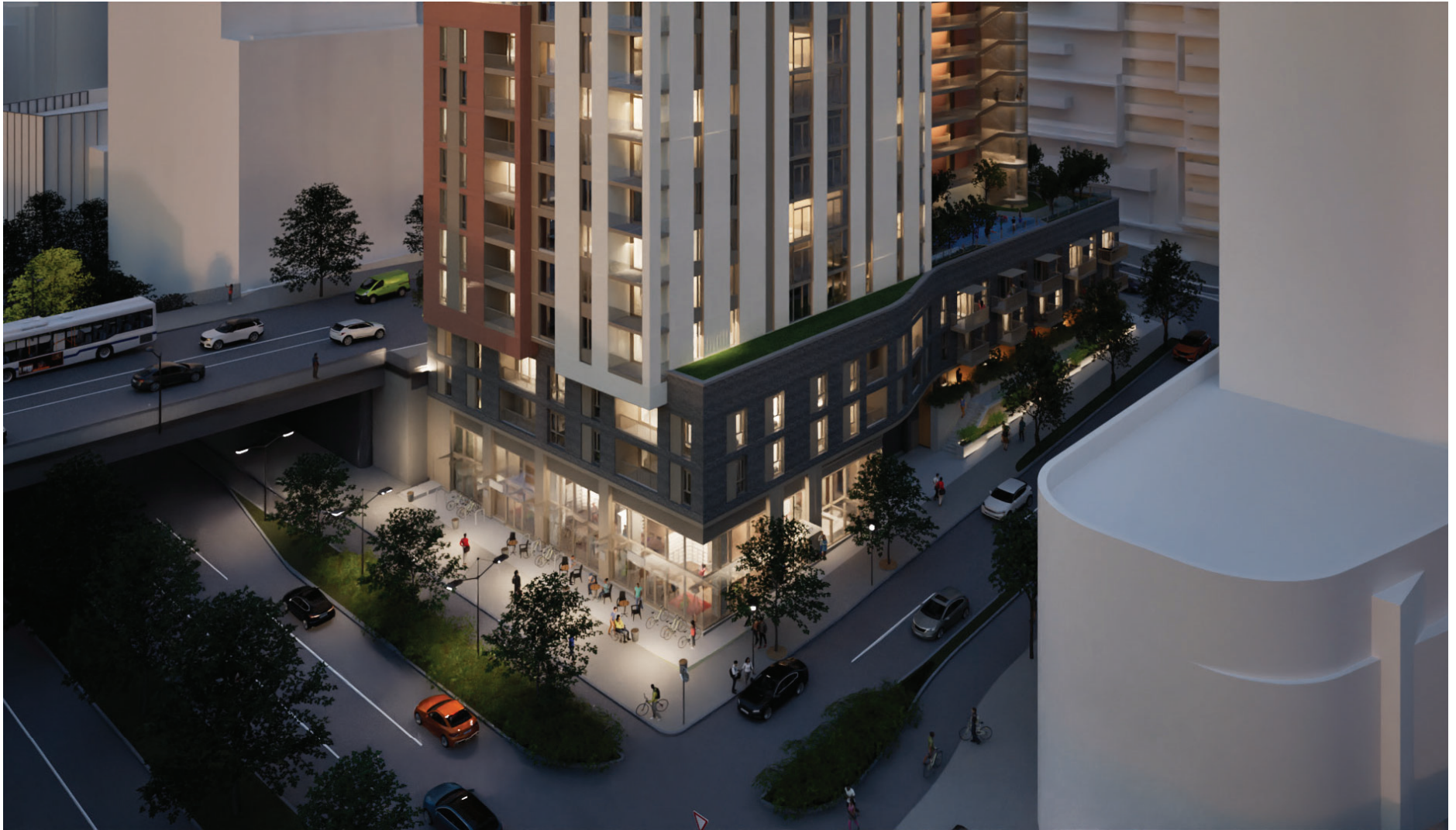
View of the southeast corner of the project site, at Pacific and Rolston Streets. While the east elevation along Rolston Street encroaches into the required 3 m setback from the SRW, the south elevation, along Pacific gives back some sidewalk space to the public realm by setting back an additional 1.5 m along the Pacific Street CRU.
