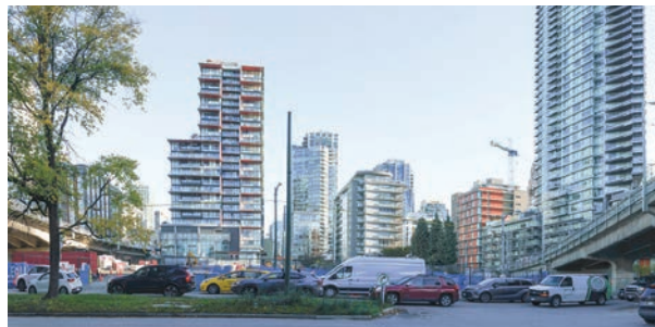
View of the site looking north from Pacific Street
