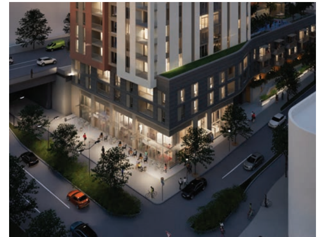
The Pacific Street elevation is set back further than required by policy, providing additional public open space.
