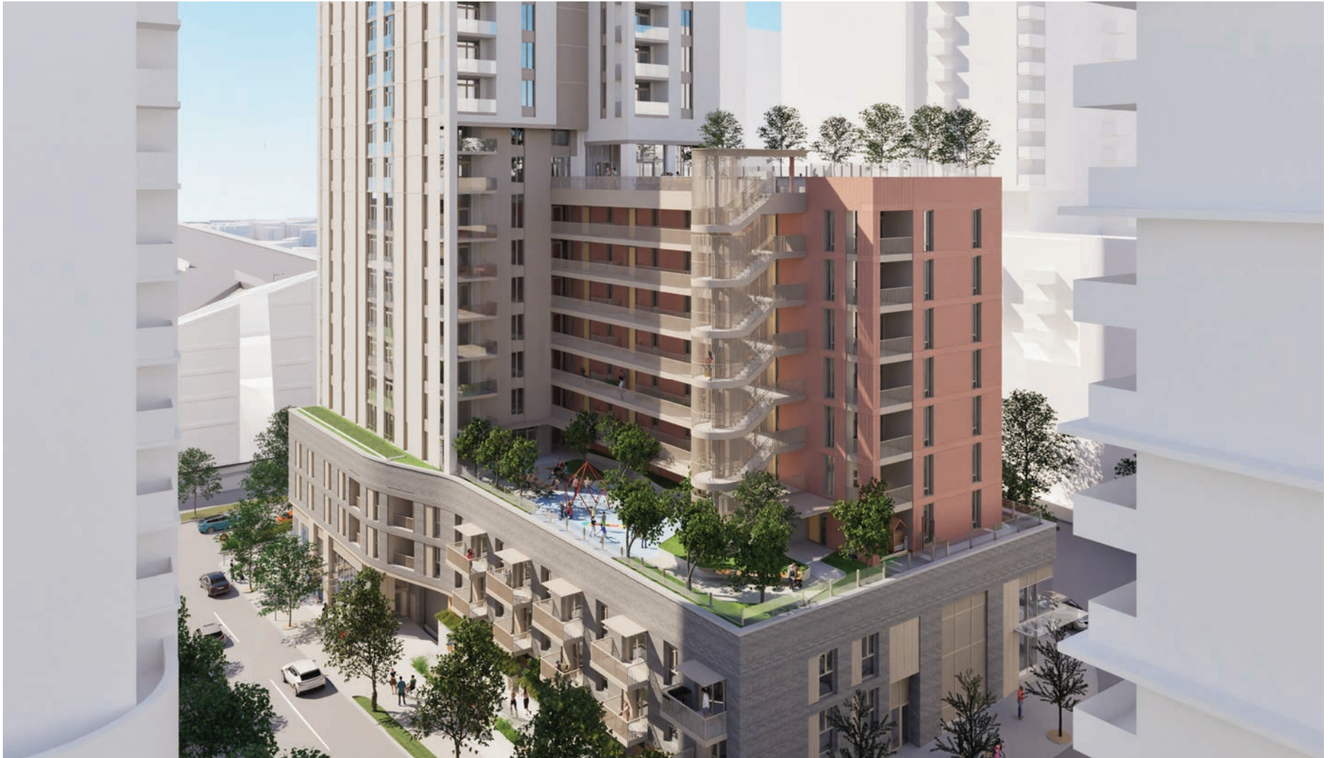
Rendered view showing the relationship between the outdoor corridors and stairs, and the way they connect the outdoor amenities at Level 5 and Level 12. The massing of Sub-area D is visible at the left of the image. The existing Rolston tower, to the North of the site, is visible at right.
