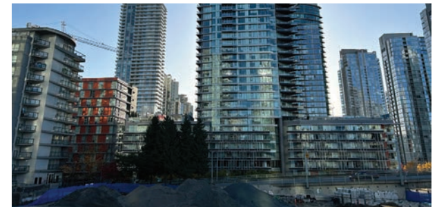
View to the east from Granville Street with the site in the foreground
