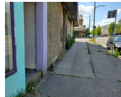
Kingsway at Site looking west
