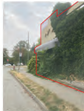
D. CAROLINA ST LOOKING NORTH
