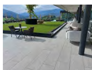
PEDESTAL PAVER SYSTEM IN LIGHT COLOUR TO REDUCE SOLAR ABSORPTION Amenity/Roof Terrace Paving
