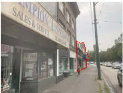
C. KINGSWAY LOOKING WEST
