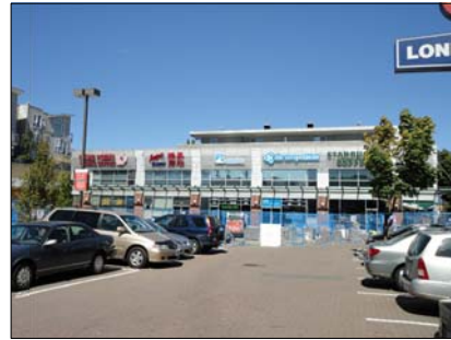
VIEW WEST FROM THE SITE
