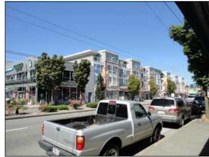
VIEW NORTH WEST FROM THE SITE
