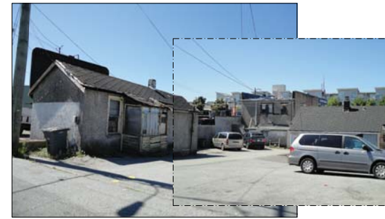
REAR OF THE SITE (VIEW WEST FROM THE LANE)
