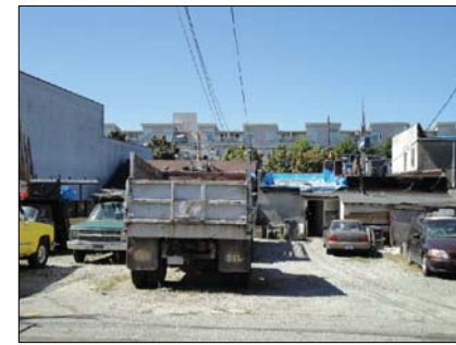
REAR OF THE SITE (VIEW WEST FROM THE LANE)
