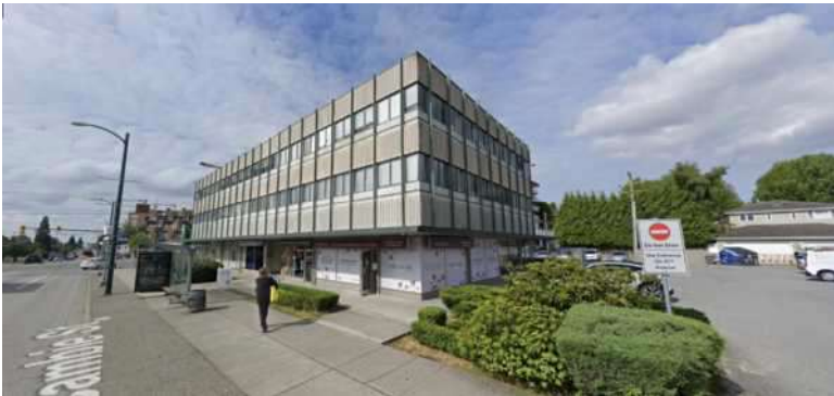
From Northeast of site, July 2022
