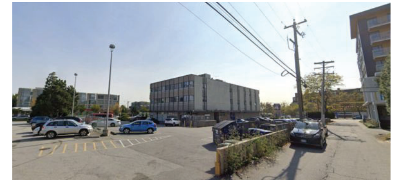
From Northwest of site, September 2020
