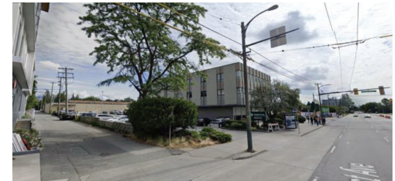
From Southwest of site, July 2022
