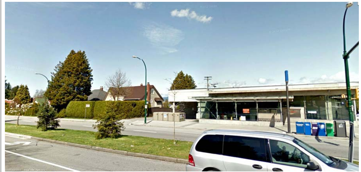
EXISTING SITE FROM SOUTH EAST
