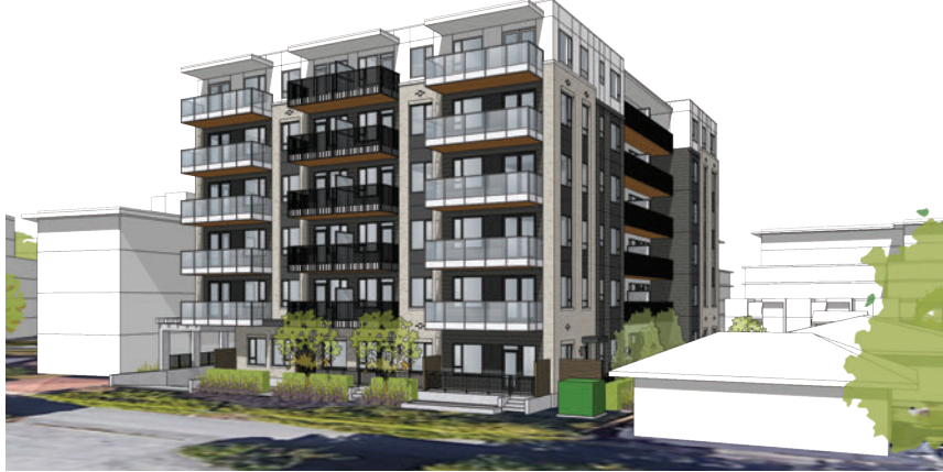
STREET VIEW FROM SOUTHWEST CORNER AT THE LANE
