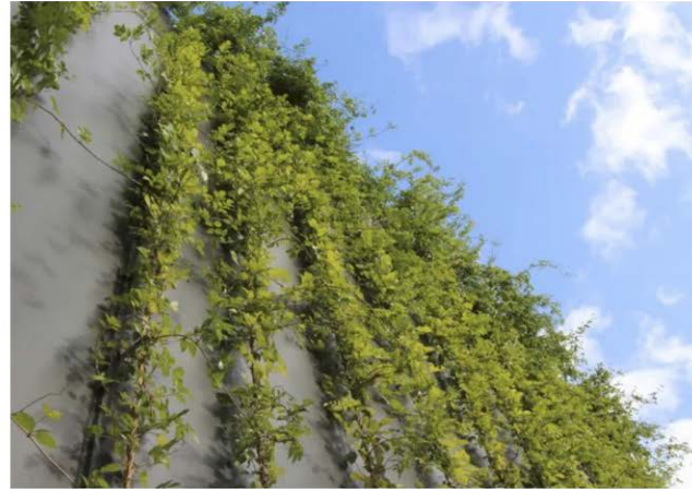
Jacob Wire System for Facade Vines
