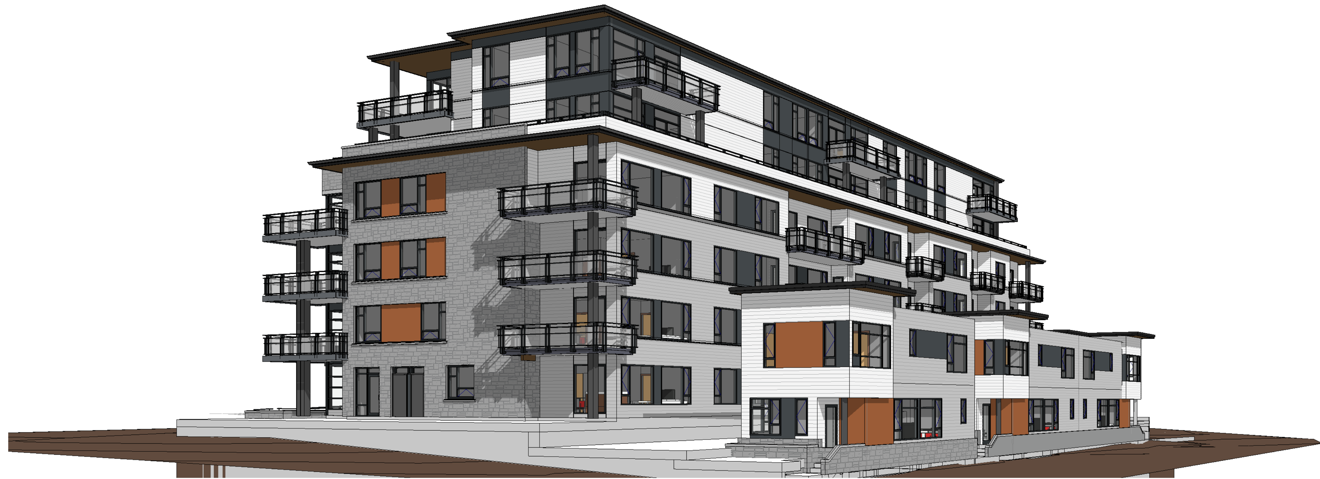
1 VIEW FROM NORTHWEST CORNER
