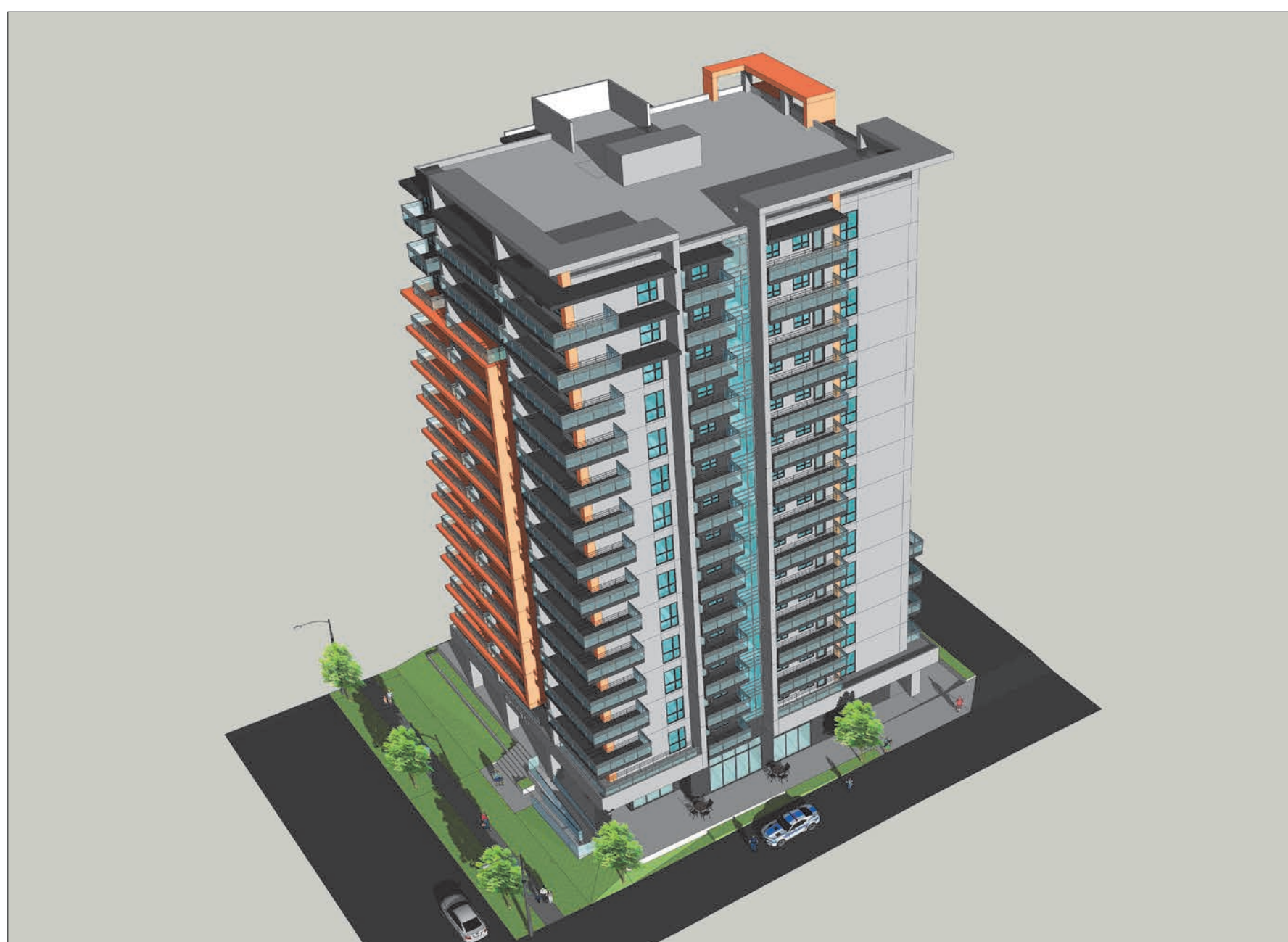
NORTHWEST TOP VIEW
