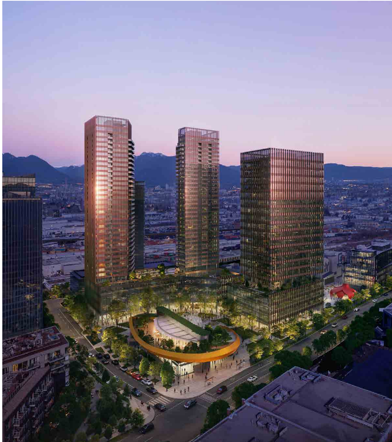
Aerial view of project looking North-East
