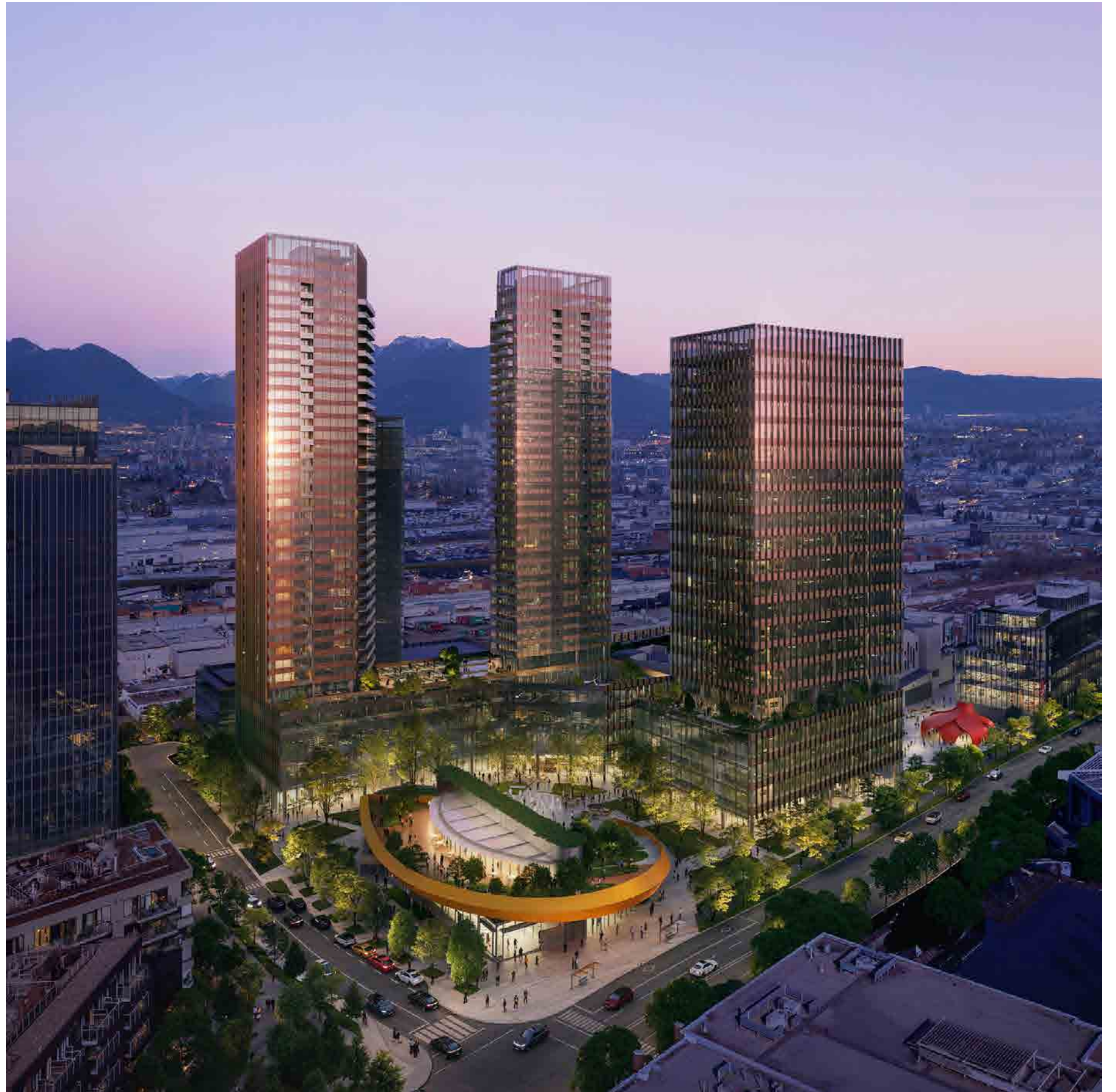
Aerial view of project looking North-East
