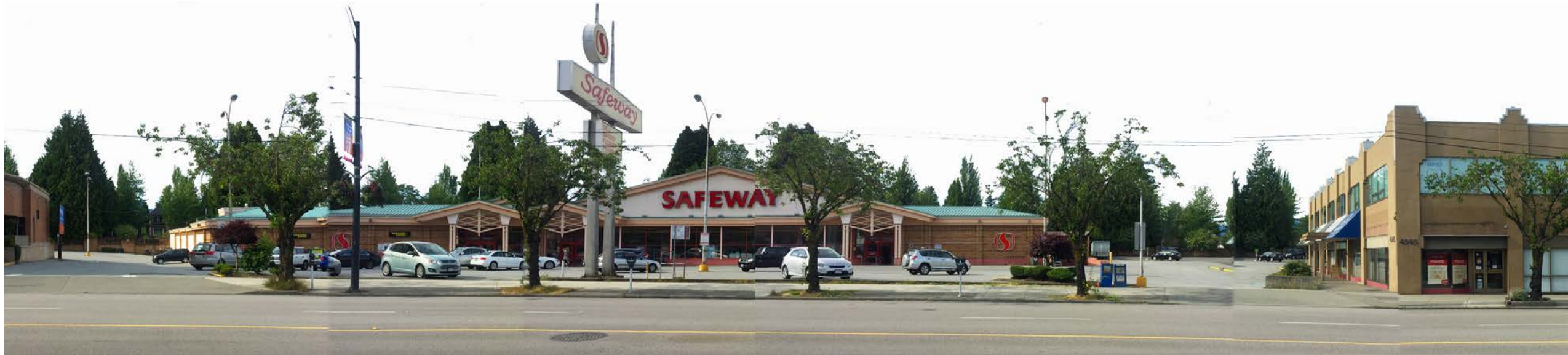
STREETSCAPE ALONG WEST 10TH AVENUE, SHOWING PROJECT SITE
