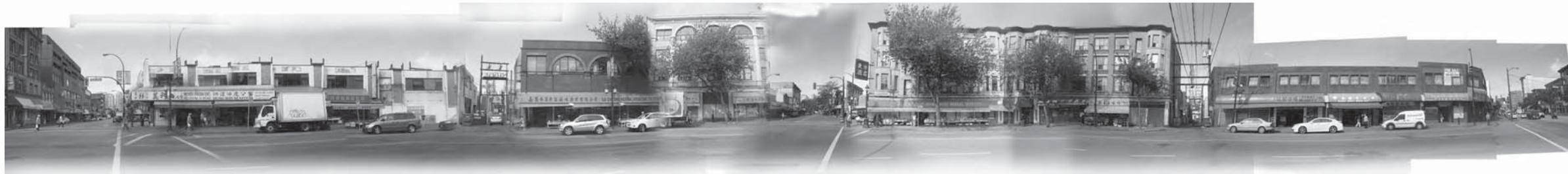
2 GORE STREET LOOKING WEST
