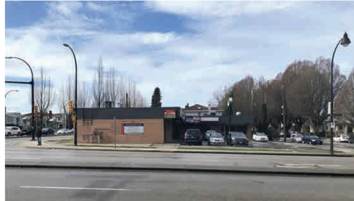
VIEW OF SITE FROM KNIGHT STREET
