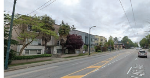
3 | SUBJECT SITE FROM WEST 4TH AVENUE TOWARDS EAST
