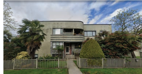
6 | SUBJECT SITE FROM ALMA STREET
