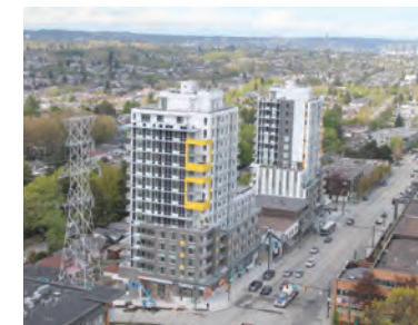
13. Looking southwest across Boundary Road and East Hastings.
