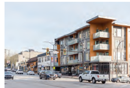
12. View from corner of East Hastings and Boundary Road looking southeast.
