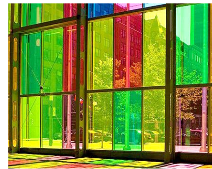
12. Coloured Glass Curtain Wall
