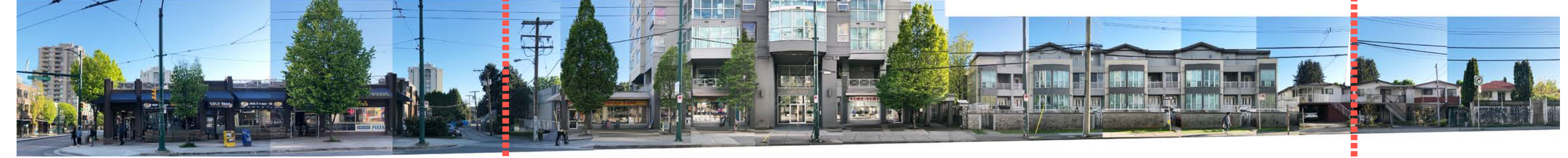
EXISTING VANNESS AVE STREETScape
