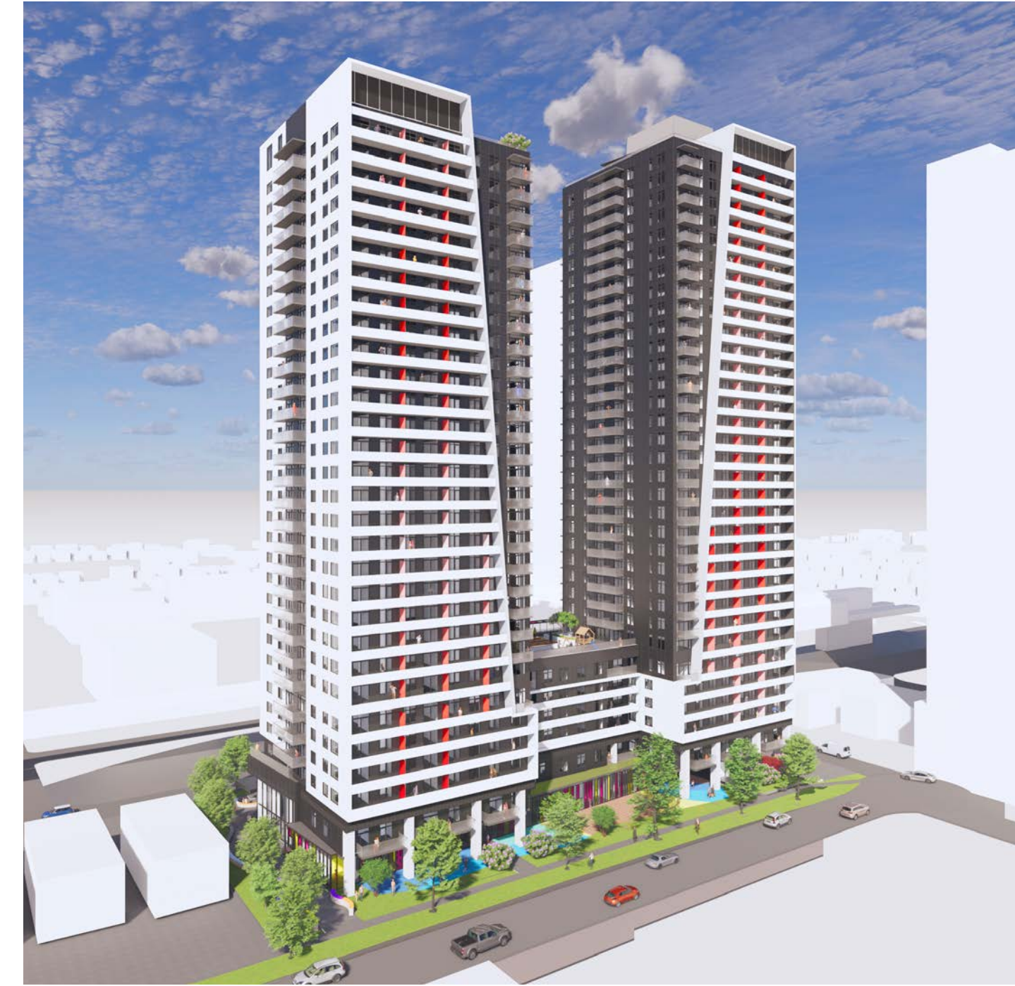
OVERALL VIEW FROM SOUTHWEST
