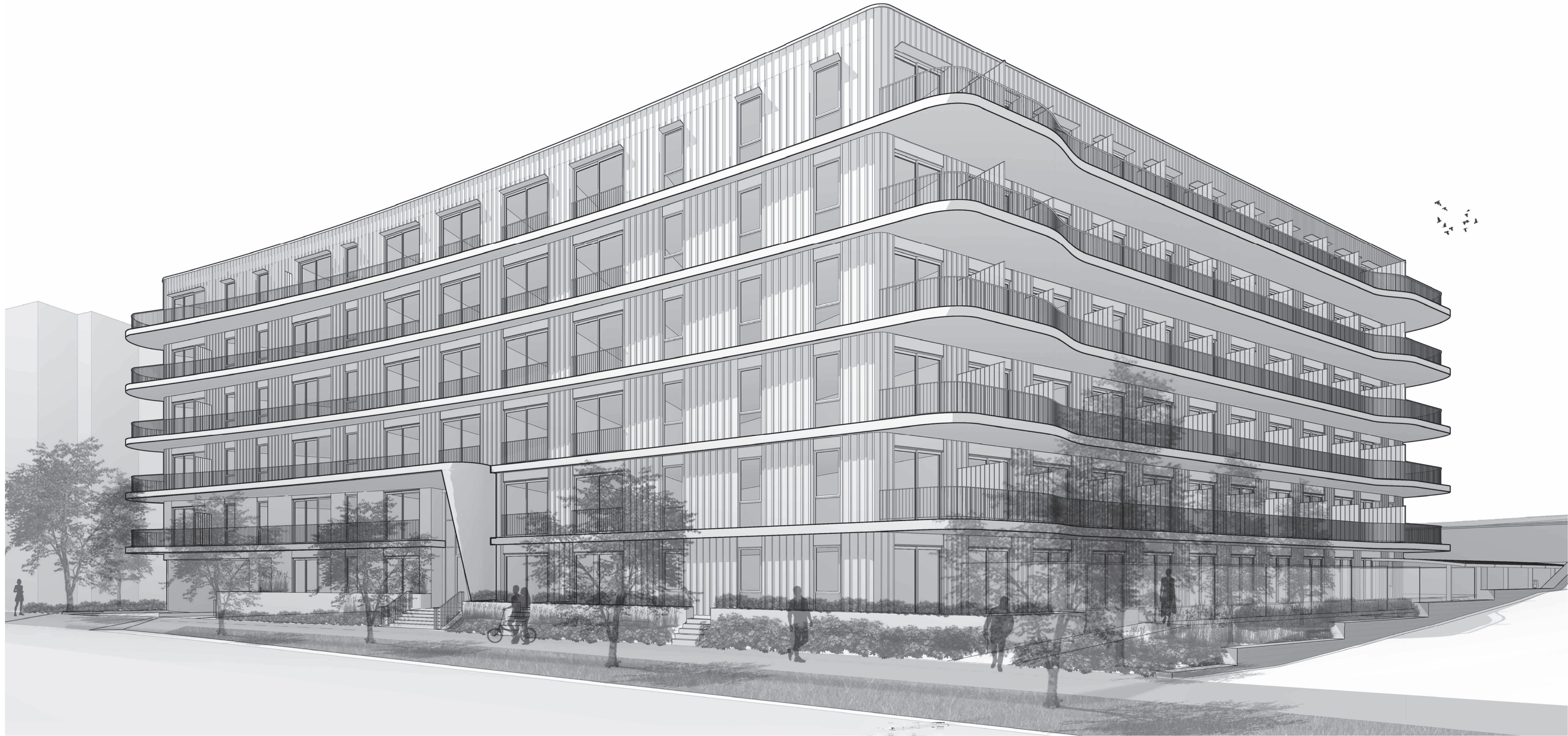
VIEW FROM NORTH EAST CORNER
