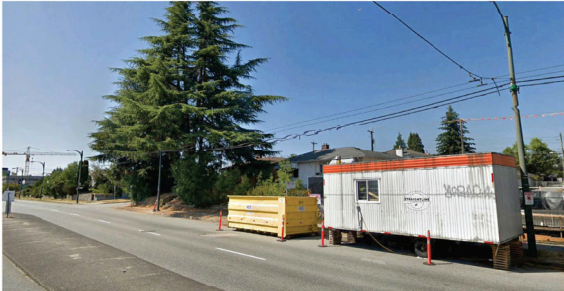
View looking North West from W41st Ave
