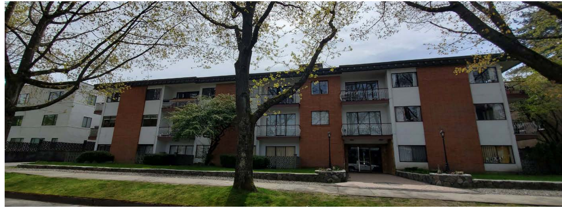
A. View of north-west corner of the site
