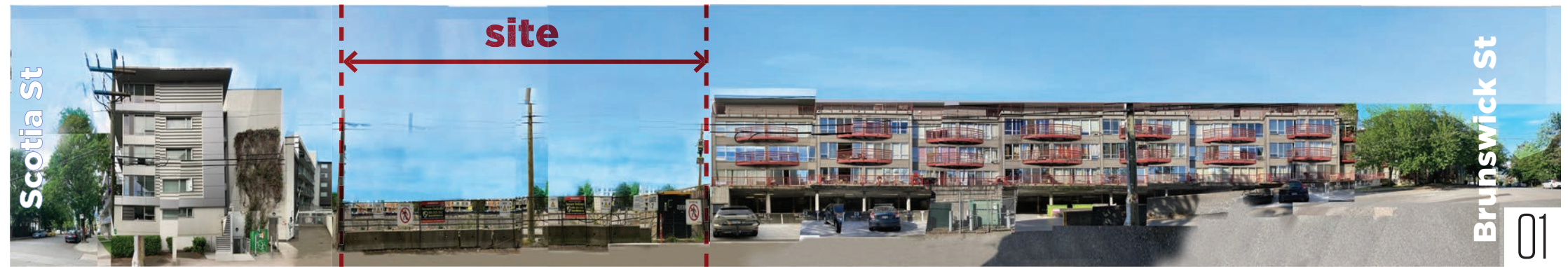
View looking north from the laneway
