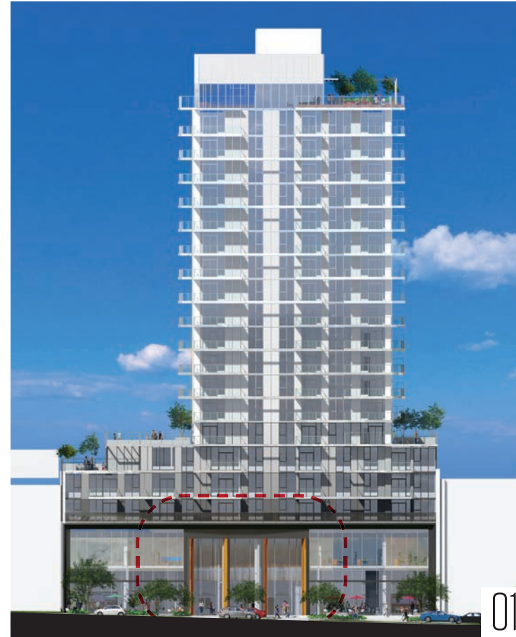
North elevation - winged lobby entrance
