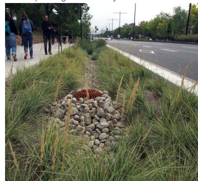
Rainwater infiltration gardens along east 14th street
