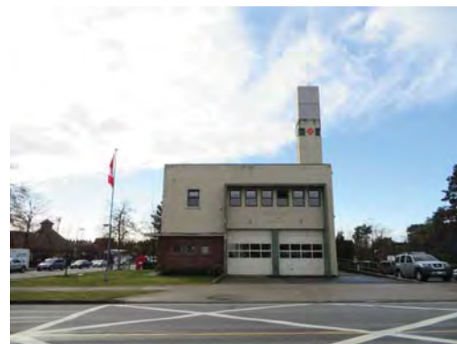
7 54th ave. looking south
