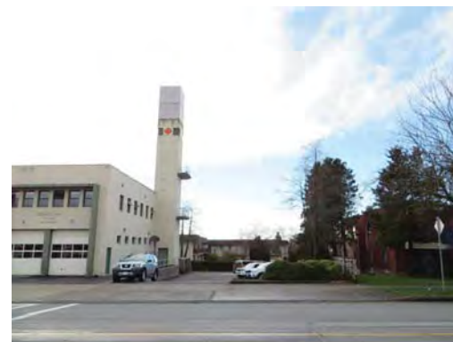
8 54th ave. looking south
