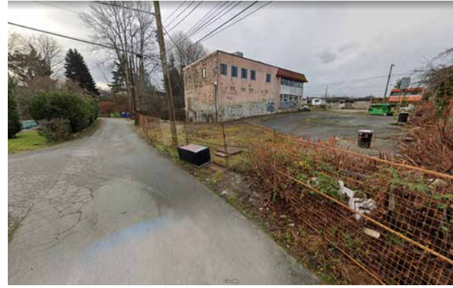
VIEW TOWARDS SW
