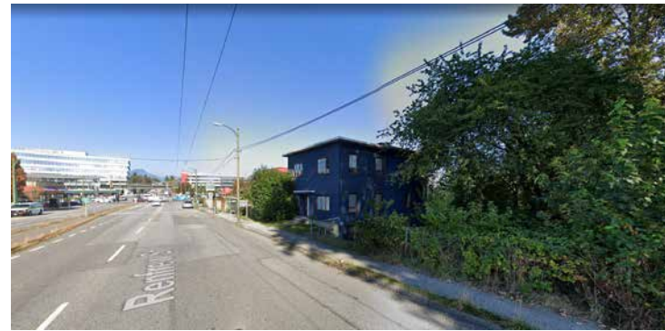
VIEW TOWARDS NW
