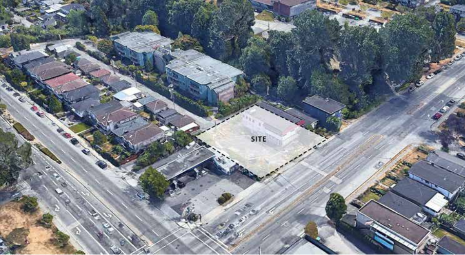
SITE - VIEW LOOKING TOWARDS SOUTH-EAST
