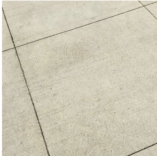
BROOM FINISHED CONCRETE
