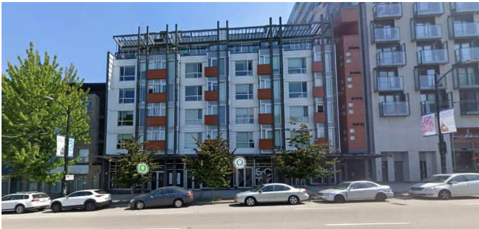
8 - Kingsway (Facing East) - Mid Block
