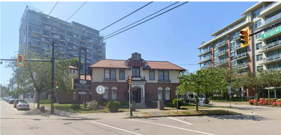
10 - East 11th Avenue (Facing South) - East Corner
