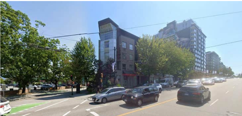
7 - Kingsway (Facing East) - North Corner
