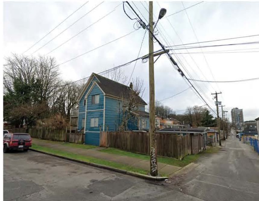
B. View of north-east corner of the site
