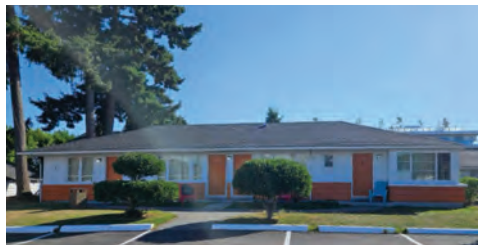
2400 Court Motel, typical bungalow
