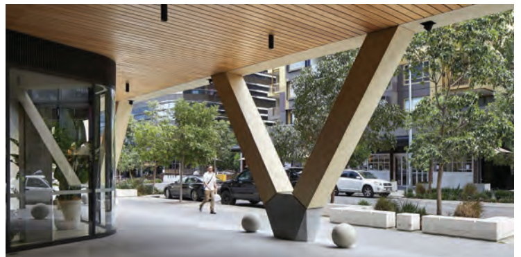
concrete and glulam 'V' column arcade and storefront windows
