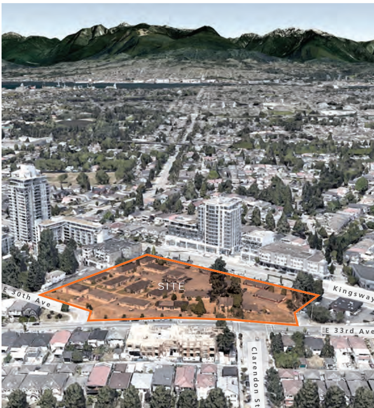
site aerial looking north
