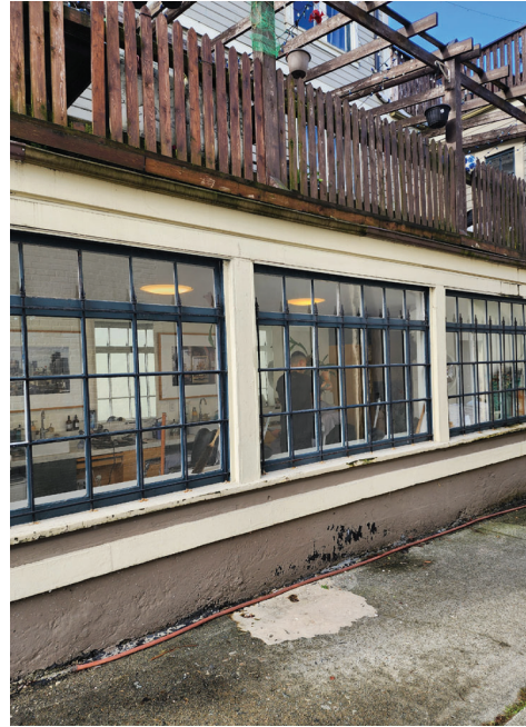
SERVICE LANE LOOKING WEST
