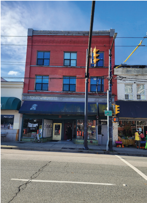
MAIN ST. LOOKING WEST - BROADWAY ROOMS
