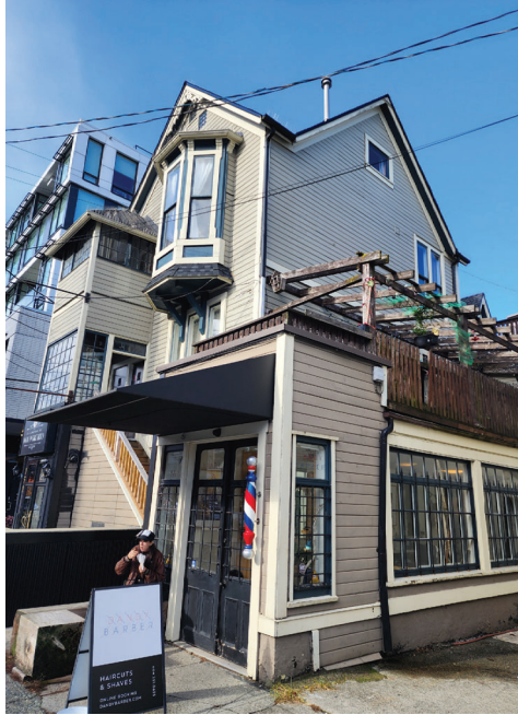
SERVICE LANE LOOKING WEST
