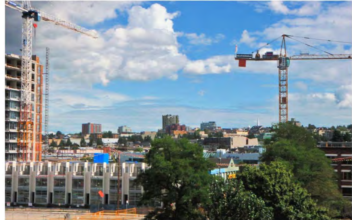
16 view from south end of Cambie bridge
