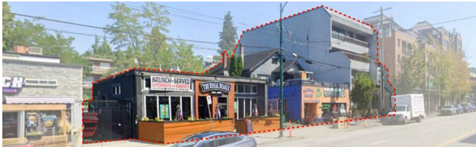
VIEW OF SITE LOOKING NE FROM BROADWAY AVE.
