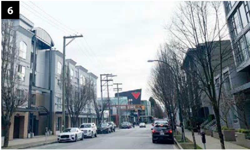
View looking East along W.7th Ave
