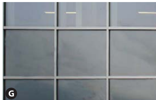
G Spandrel Glass Colour: Grey Layered behind the curtain wall to ensure privacy for the occupants.
