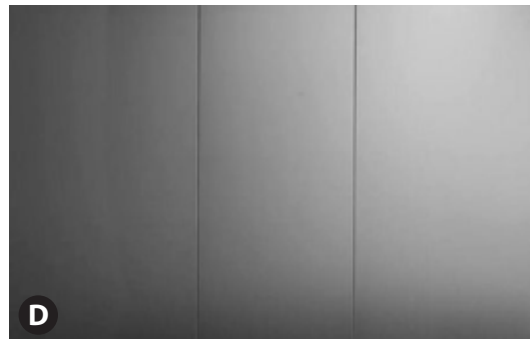
D Exterior Metal Panel Colour: Grey/Silver To accentuate the tower's slender proportions and provide solar shading.
