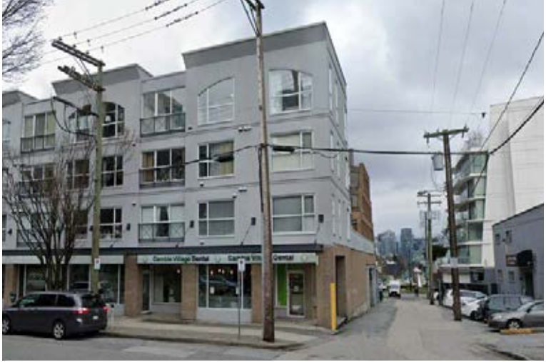
Existing residential building to the west
